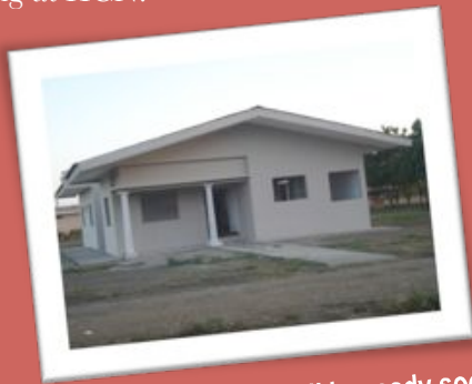
The new girls home will be ready soon!
